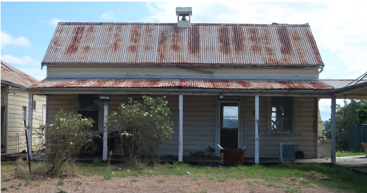
Photo 3-17 The front east elevation of the kitchen building
