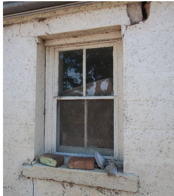
Photo 3-10 A typical original sash window in the east facade
