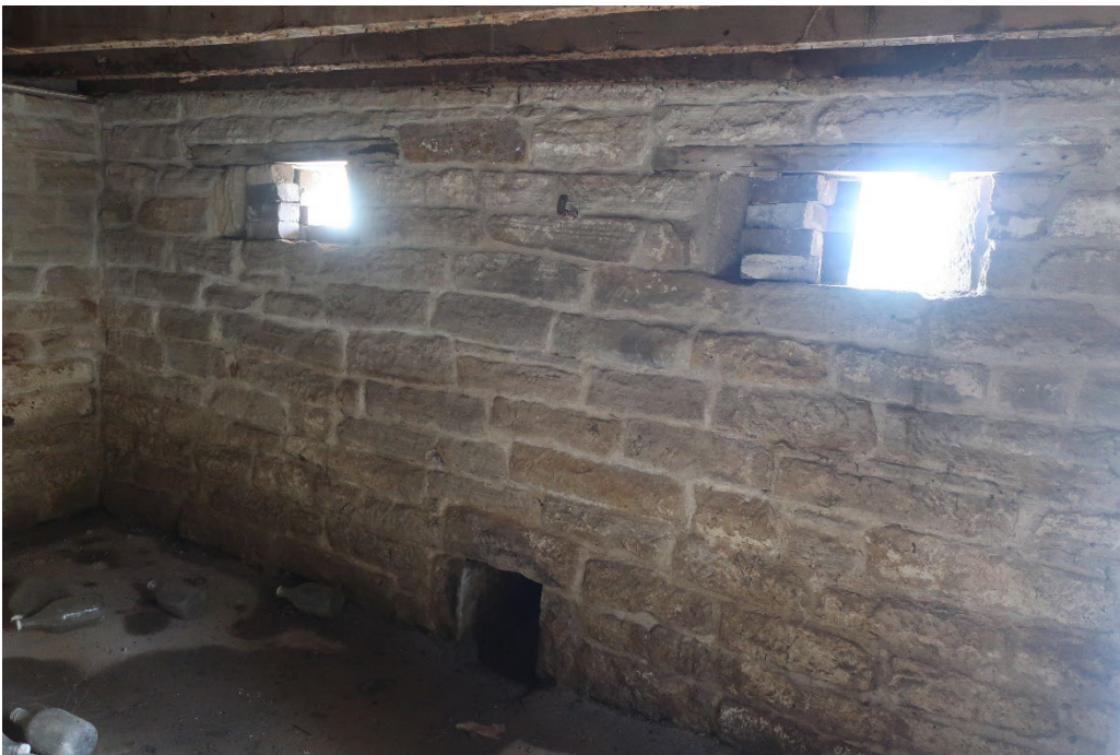
Photo 3-8 The basement cool room under the west end of the homestead
