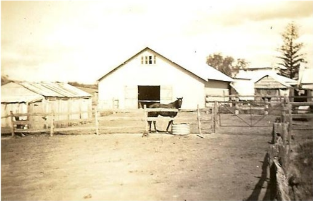
Figure 2-8 Southwards view c1960 showing the post-war stable, and the homestead with pop-up extension behind. The slab hut with corrugated steel roof on the left is long gone.
