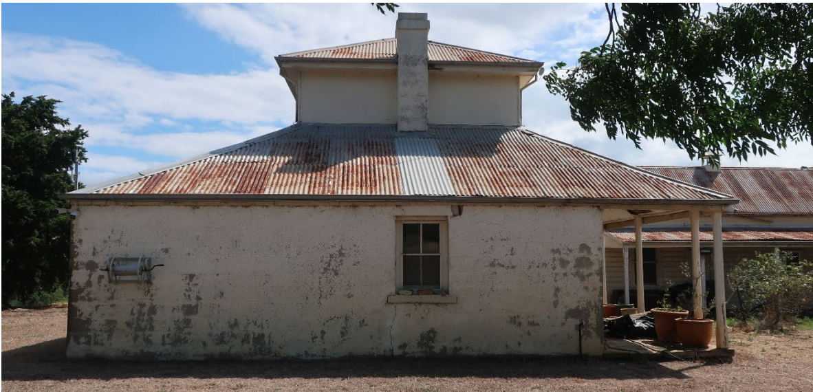
Photo 3-7 The east elevation of the homestead
