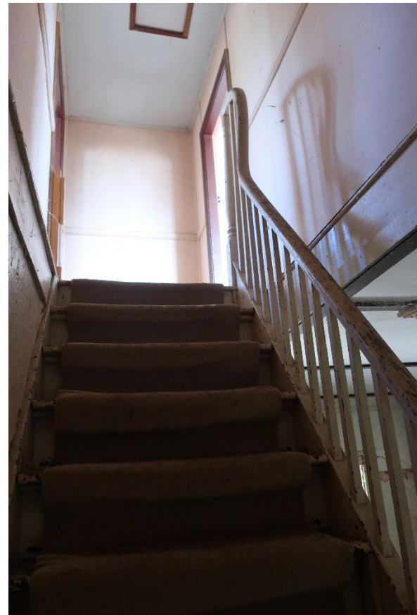
Photo 3-12 Georgian goose-necked balustrade at the top of the stair
