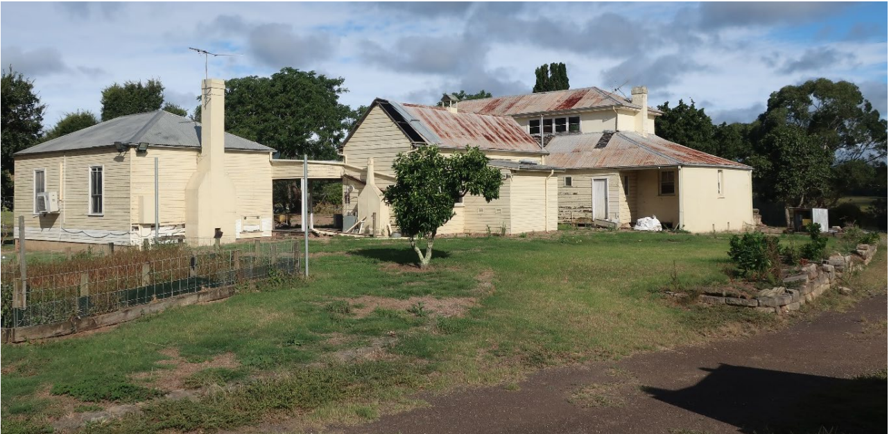
Photo 3-2 The Meadowvale group looking south-east, showing the 1990s neo-Victorian building on the left, the kitchen building (centre) and the homestead behind and to the right
