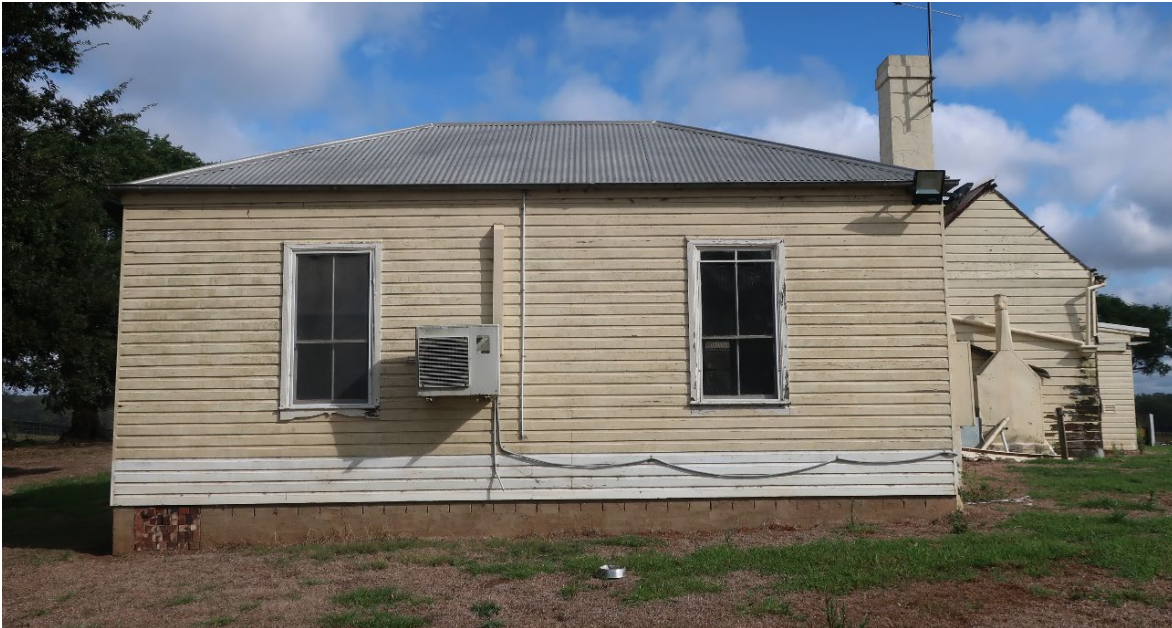
Photo 3-22 The northern façade of the northern cottage, the kitchen is seen behind on the right
