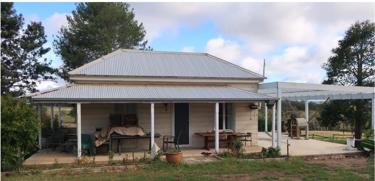
Photo 3-20 The northern front of the southern cottage
