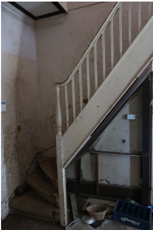
Photo 3-11 The stair is clearly original
