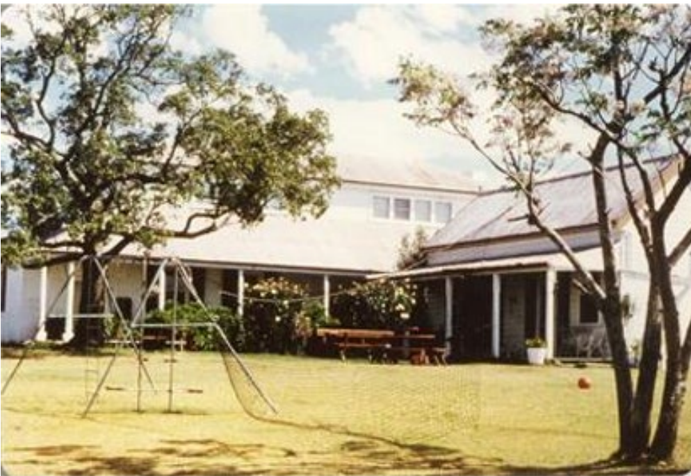
Figure 2-13 1979 southwards view of the rear of Meadowvale showing the kitchen on the right.
