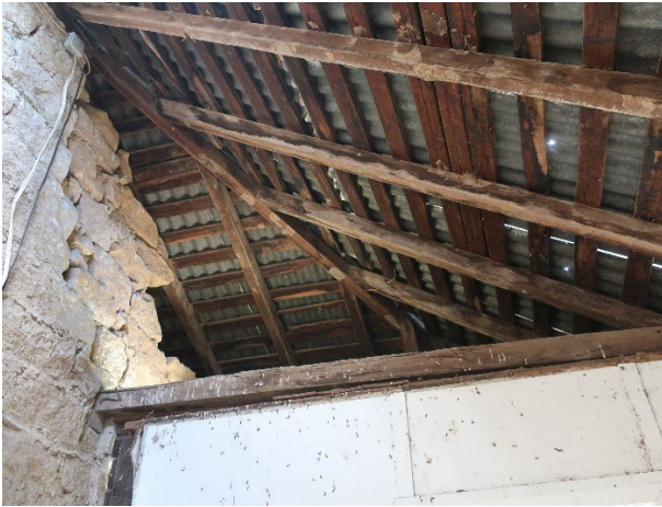
Photo 3-13 Original roof framing above the former laundry on the northern side of the homestead
